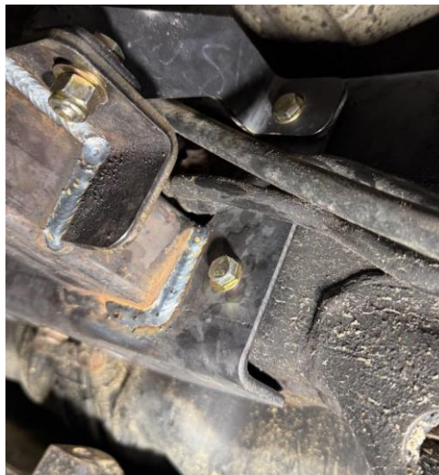
Completed driver-side mounting area
